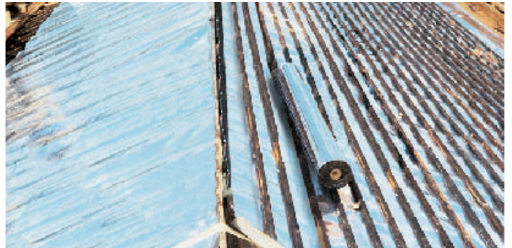
AHI foil installed under battens.
