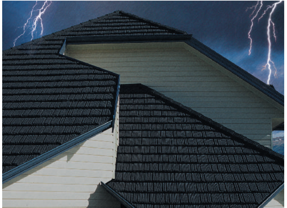
Well earthed building undamaged by passage of lightning.
