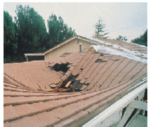
These cement shakes slipped causing sub-structural damage
