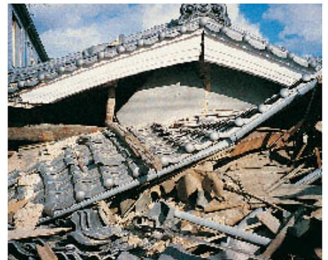
Traditional clay tile roofs are inevitably heavy weight and cause structural damage in Earthquakes
